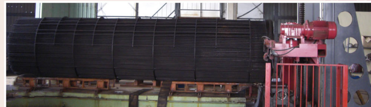
冷凝管切削工廠實景 Cutting heat exchanger pipe
